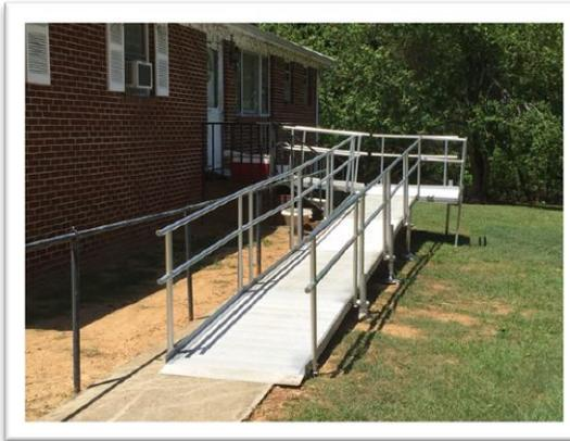
aluminum ramps to those needing a ramp for short, indeterminate periods of time. These ramps can be installed by two people in a couple hours and can be removed when no longer needed, to be set up again elsewhere. Currently we have over 130 sets of these
